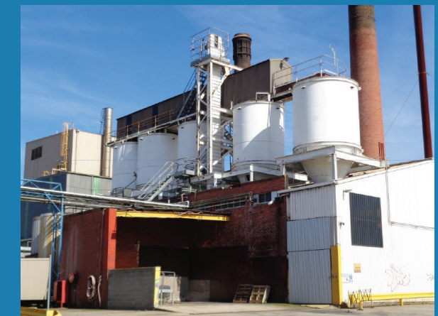
Boilers and Coal Handling
